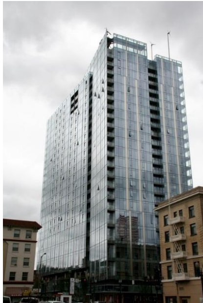
Figure 8 Twelve West building, Portland, USA [51], permission for use authorized by Wikimedia Commons.
