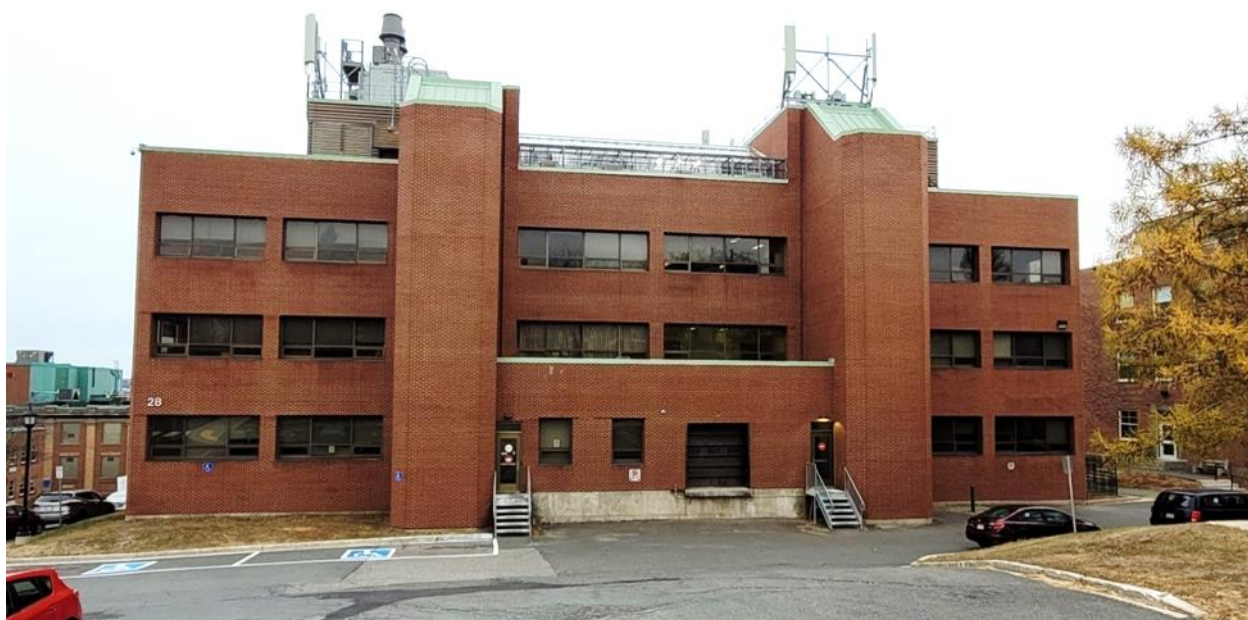
Figure 1 IUC Forestry Building, a three-story steel-frame institutional building.
