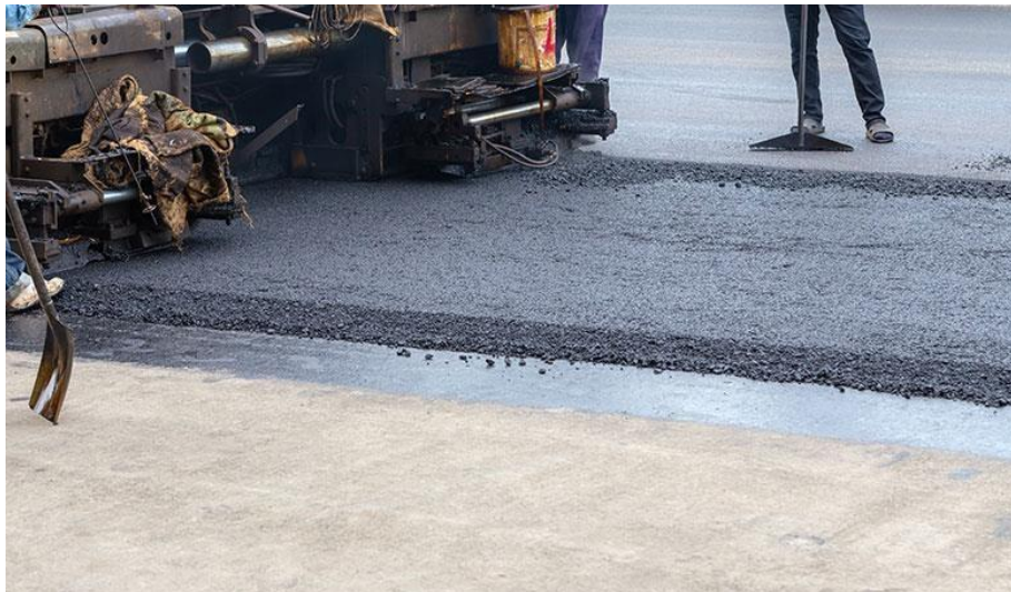
Figure 7 Typical pictorial representation of Asphalt as a civil Engineering material. Source [2].
